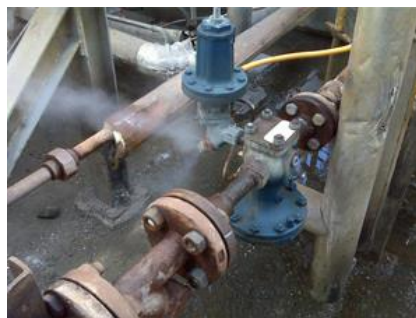
Figure 5.10 Steam leaks
