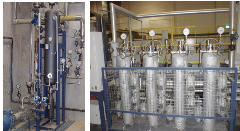
Figure 5.12 Steam condensate collection and recovery
