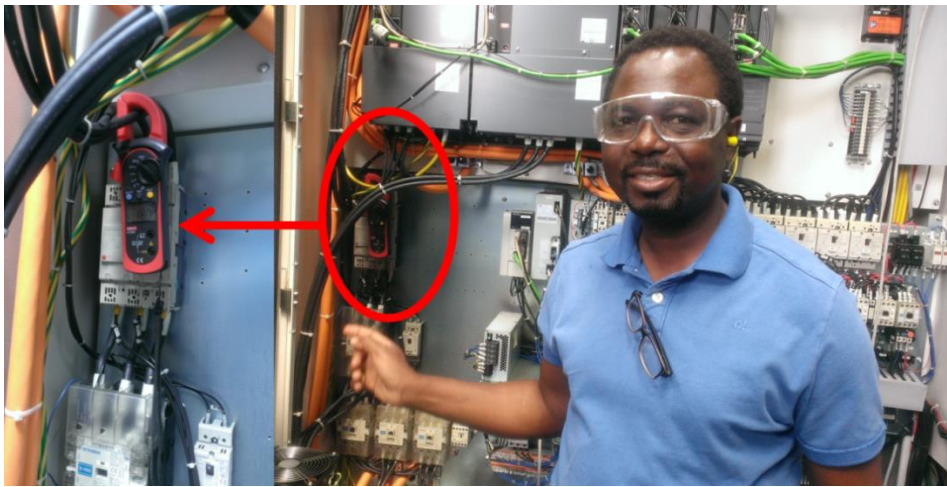
Figure 7-8 Clamp meter connected to the 3-phase source to measure the input current on the load
