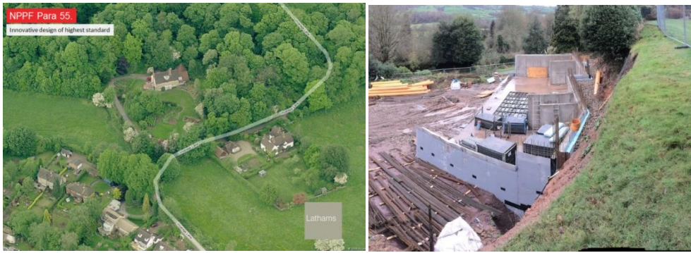
Figure 1: (a) Aerial View - Site Location; (b) Site build progress
