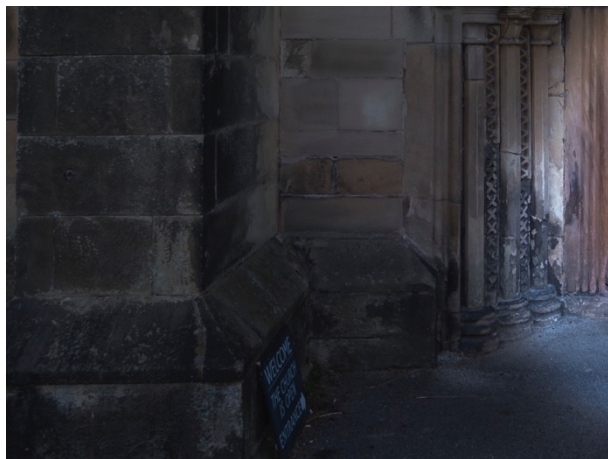
Figure 78 Test #2 Mark Hall
