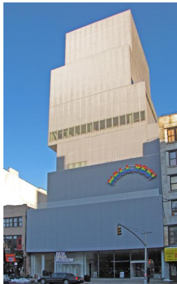
Fig 1.9 SANAA's New Museum building, Bowery, New York City. © Stu pendousmat
