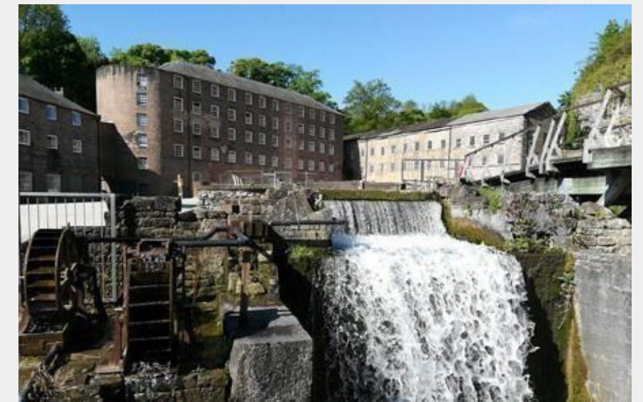
Cromford Mills existing watercourse and wheels
