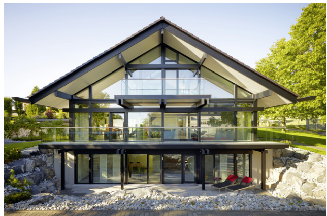
Figure 1. An example of post and beam systems (also known as stick built in the UK)
