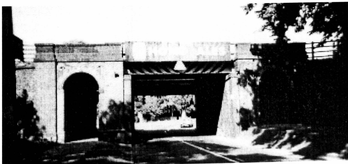
Figure 4.5: Bridge at Barrowby Road, Grantham.
