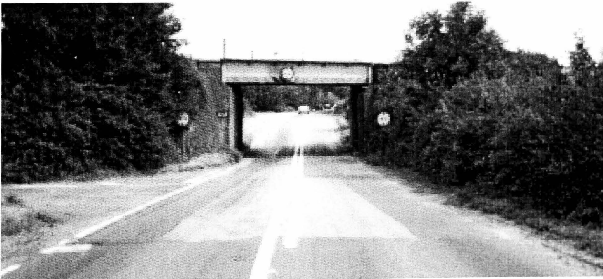
Figure 1.1: Example of a girder bridge
