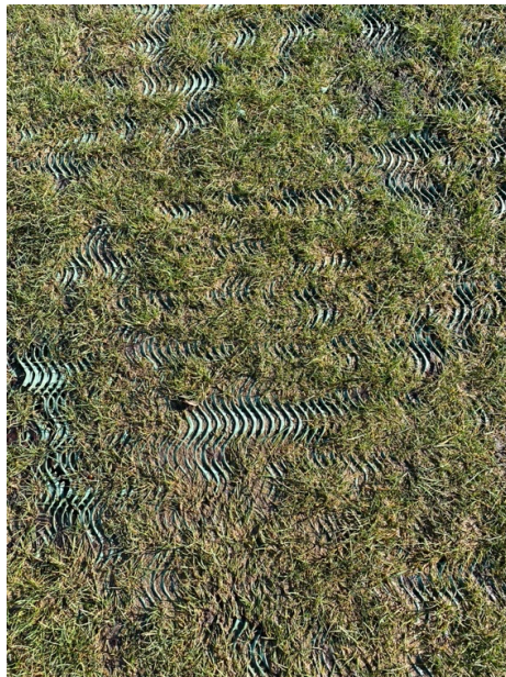
Figure 73. Plastic ground reinforcement matting installed at the site of Timber festival. Author's photograph.
