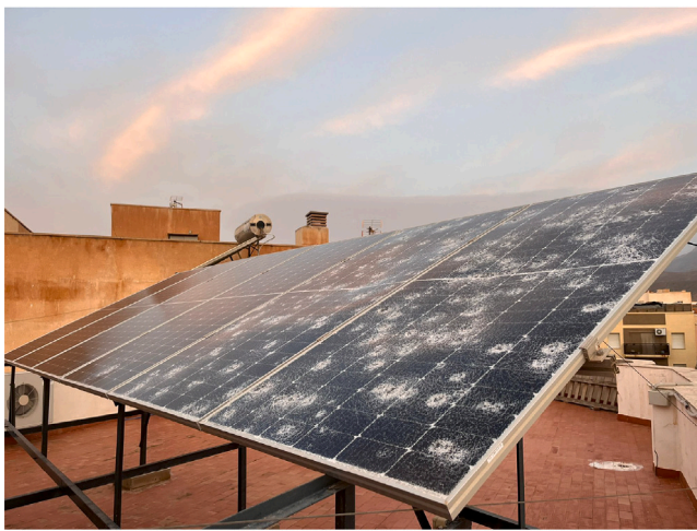
Fig. 8. Solar panels after a hail storm.
