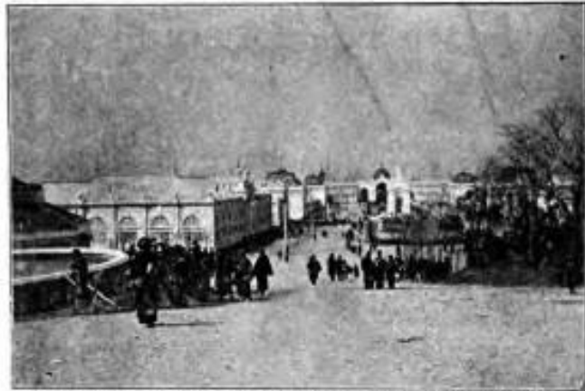
VIEW OF THE FRONT GATE FROM FINE ART BUILDING.
