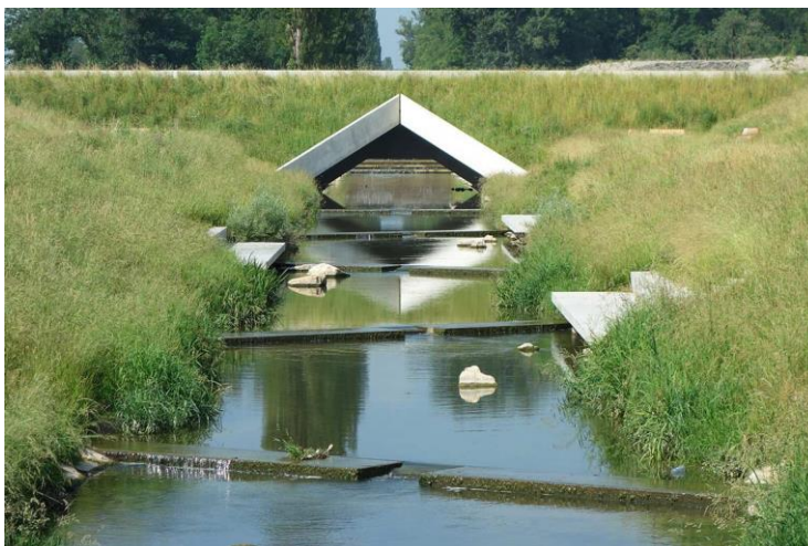
Fig. 5. Renaturation of the River Aire – Discharge area of the river still showing signs of an artificially shaped flow via a diamond-shape pattern. Courtesy © Superpositions.
