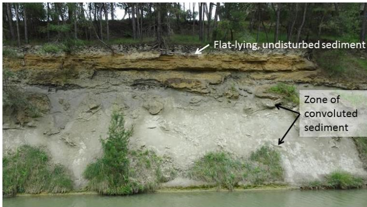
Figure 18. Canal du Midi cutting several metres high just outside the Malpas Tunnel showing convolute sediment below undisturbed, thin beds of shallow-marine sandstone
